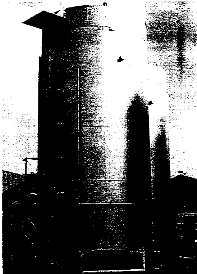
Figure 13.2 Typical Enclosed Ground Flare
