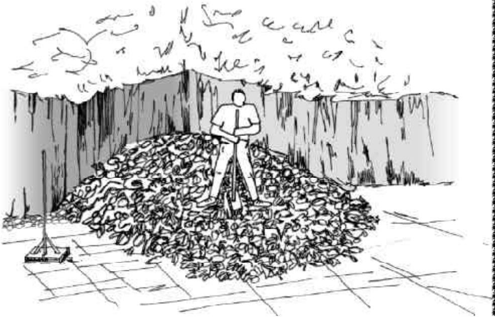
Figure 7.16 Compacting MSW with a hand tamper
