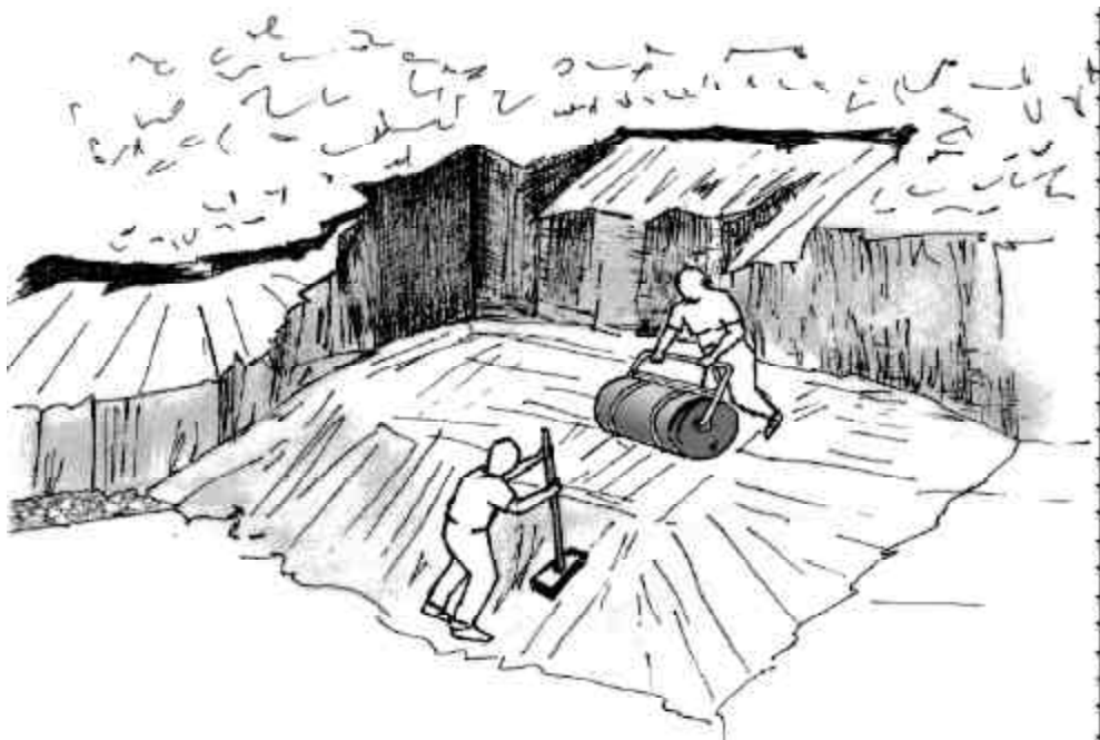
Figure 7.19 Compaction of the first finished cell with roller and hand tamper
