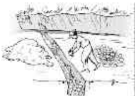
7. Construction of internal drainage
