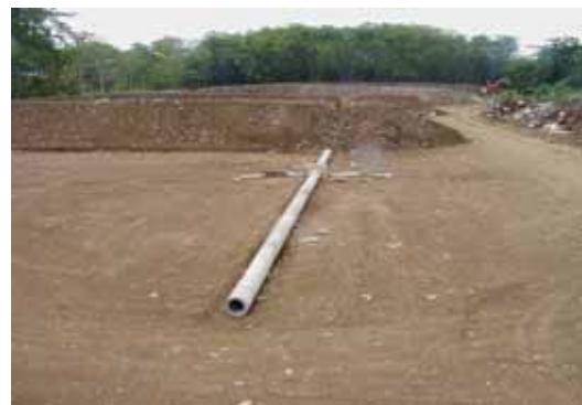
Photo- 16: Concrete Pipe Setting
