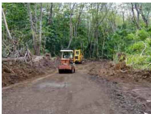
Photo- 6: Compaction & Gravel Paving
