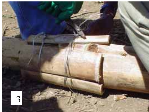
Photo- 15: Bamboos as Substitute Material for Pipes
