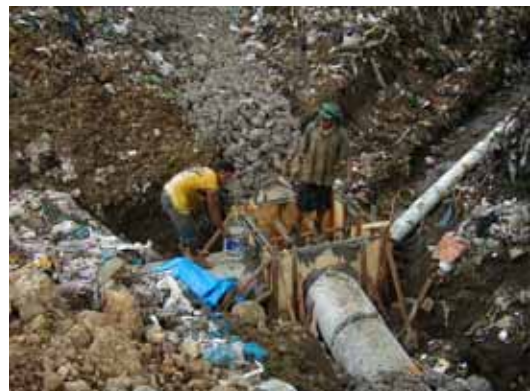
Photo- 22: Installation (in-situ concrete) of Connection Pit in Deep Waste Layer
