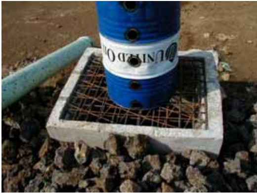
Photo- 23: Vertical Gas Venting Pipe installed on Pipe Connection Pit
