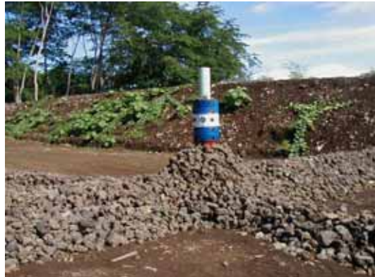
Photo- 23: Vertical Gas Venting Pipe installed on Pipe Connection Pit
