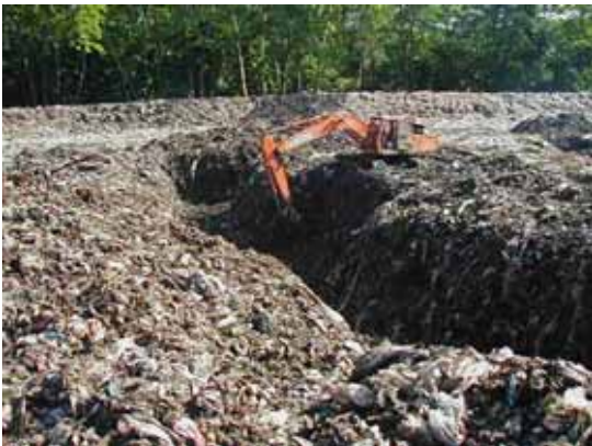
Photo- 18: Excavation of Trench at Deep Waste Layer
