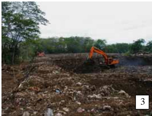
Photo- 13: Sequence of Enclosing Bunds Construction
