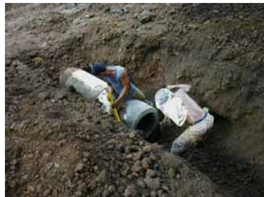
Photo- 12: Diversion Pipe Setting
