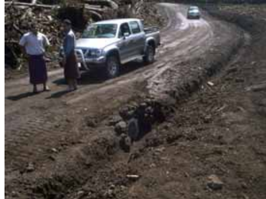
Photo- 9: Side Ditch with Road Crossing Culvert
