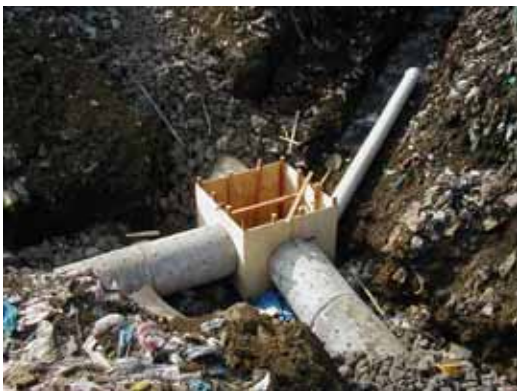
Photo- 22: Installation (in-situ concrete) of Connection Pit in Deep Waste Layer
