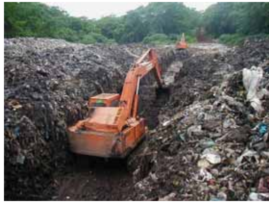
Photo- 18: Excavation of Trench at Deep Waste Layer
