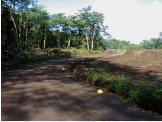
Photo- 8: Side Ditch with Curb Stone
