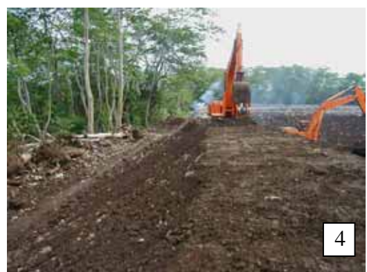
Photo- 13: Sequence of Enclosing Bunds Construction
