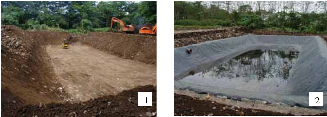
Photo- 20: Leachate Retention Pond
