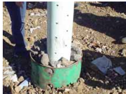
Photo- 24: Vertical Gas Venting Pipes at Landfilled Area
