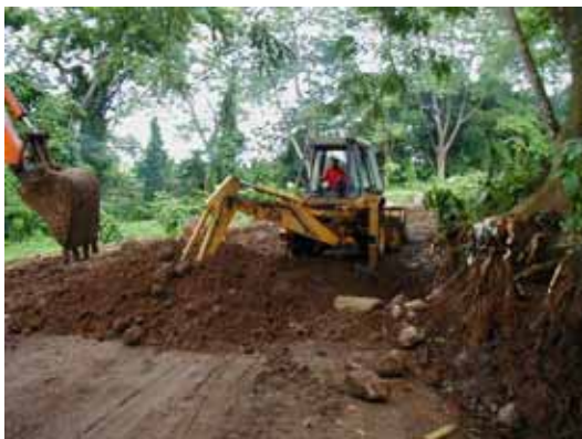
Photo- 11: Excavation of Trench
