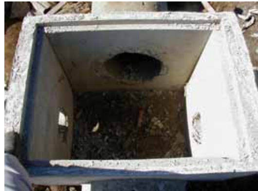
Photo- 21: Pipe Connection Pit
