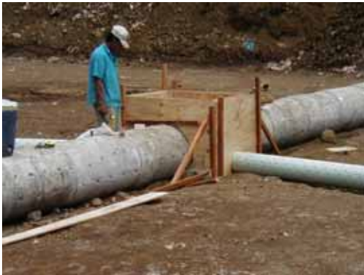
Photo- 21: Pipe Connection Pit
