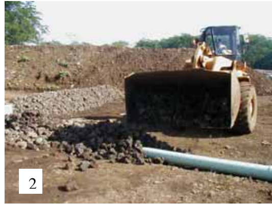
Photo- 17: Installation of Pipes and Protective Gravel Layer
