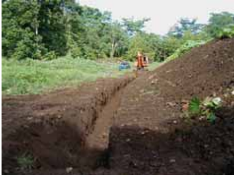
Photo- 10: Perimeter Drain Excavation
