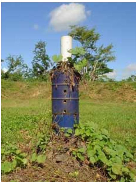
Photo- 24: Vertical Gas Venting Pipes at Landfilled Area
