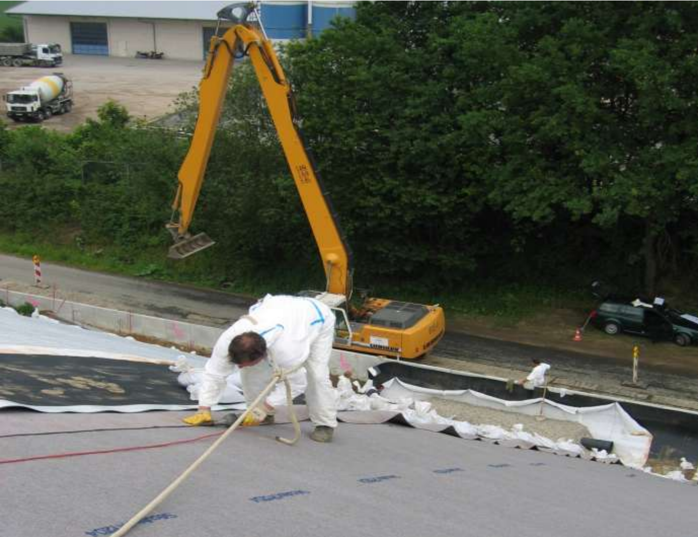
Steep inclination of cap sealing system on salt slag landfill (Furth im Wald, Germany)
