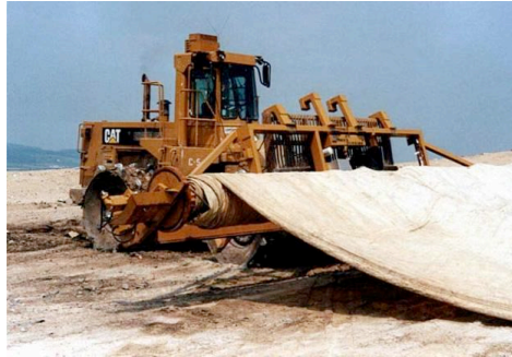
Figure 2.2. Application of Geotextile Matting
