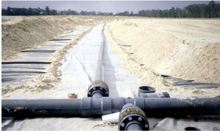
Figure 12.2. Leachate collection and conveyance system
