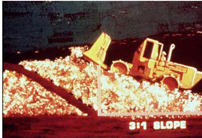
Figure 8.2. Compaction slope (3:1) of the landfill area
