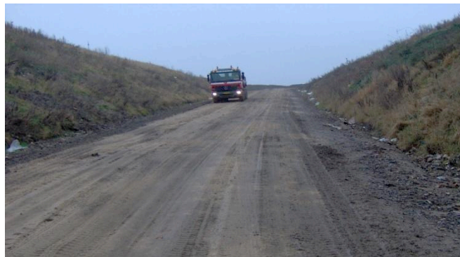
Figure 1.4. Hard-core secondary access road
