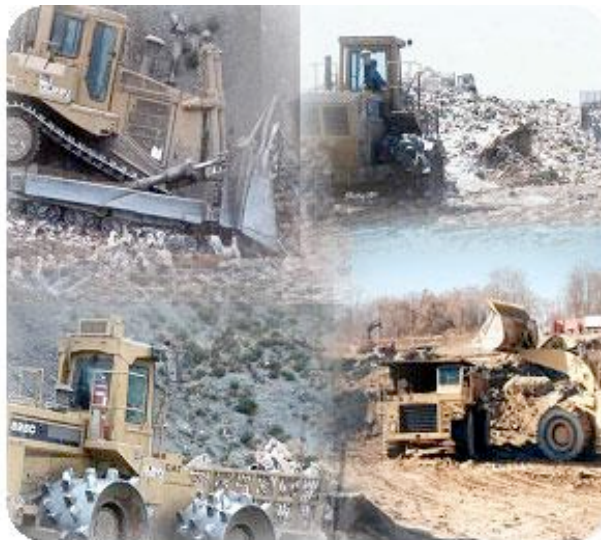
Figure 7.1. Placement of the first layer of waste
