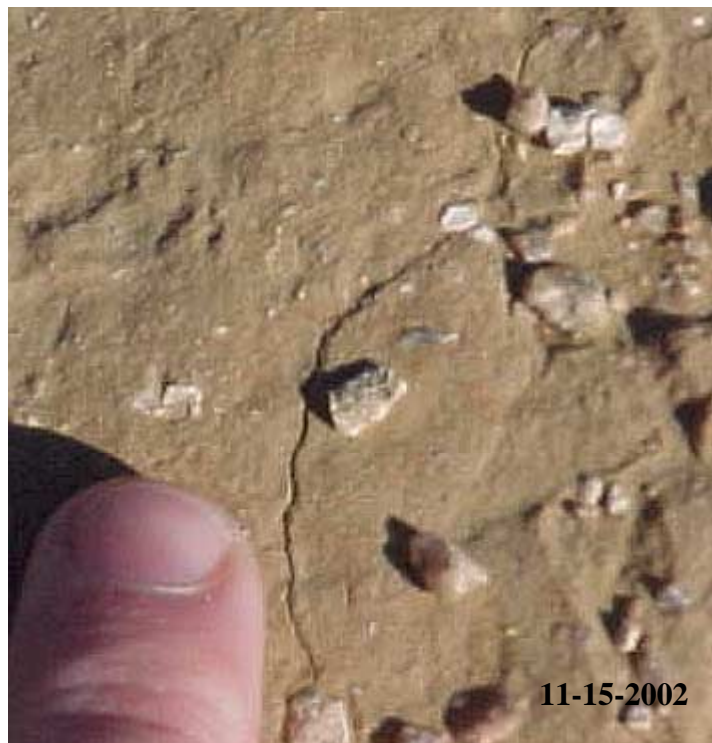
Figure 3.22. Desiccation Crack in Subtitle D Cover (Barrier Layer)
