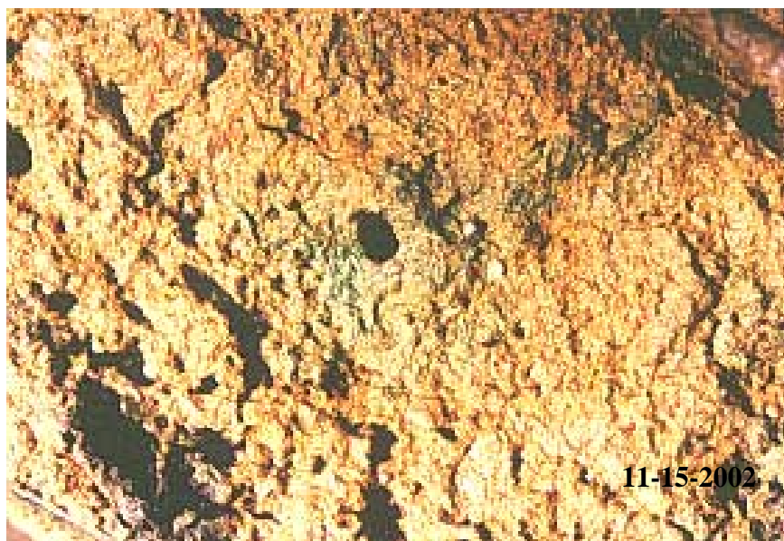
Figure 3.24. Earthworm Hole in Subtitle D Cover, Barrier Soil Layer
