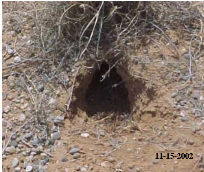
Figure 3.25. Burrowing Animal Hole on Anisotropic Barrier
