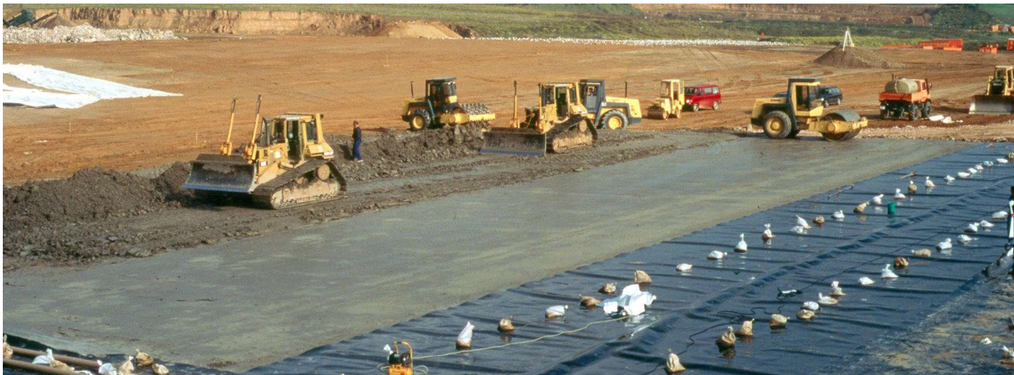
Watering, Sheep-foot compacting, levelling, smooth compacting (typical for two layers)
