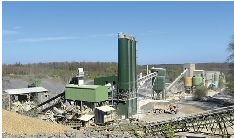
Processing of Clay and site transportation
