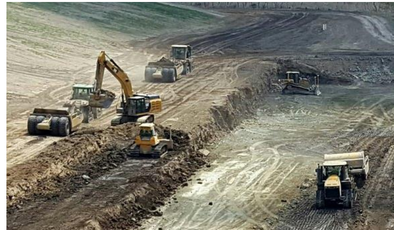
Subgrade preparation and clay spreading
