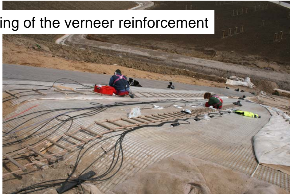
Installation of the strain gauges
